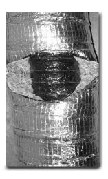
From a center of the bend cut the cotton insulation (careful not to damage the inner core!) with circular saw (blade reversed) and bend the jacket in a 45° angle (e.g. cut out a football shape piece) in both directions to achieve a 90° angle.
