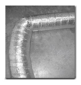
Bend the duct to desired 90° angle and tape the jacket with UL 181 B tape.
